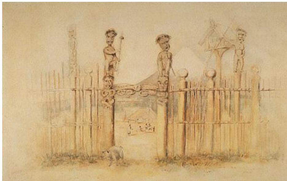
Fig. 1: Traditional Pā (village) entrance
